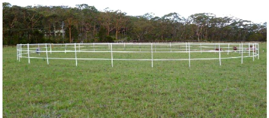
**Note; the above Round yard is 20m diameter with 30 x Fibopost 600XT 1800mm post spacing is 2.1m**
